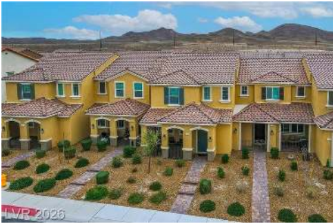
Terracotta tile roofs crown this vibrant residential row, set against a distant, arid mountain range.
