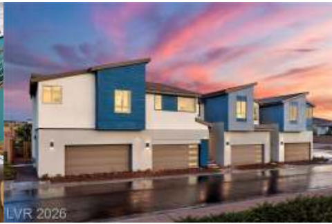
Front of Structure
